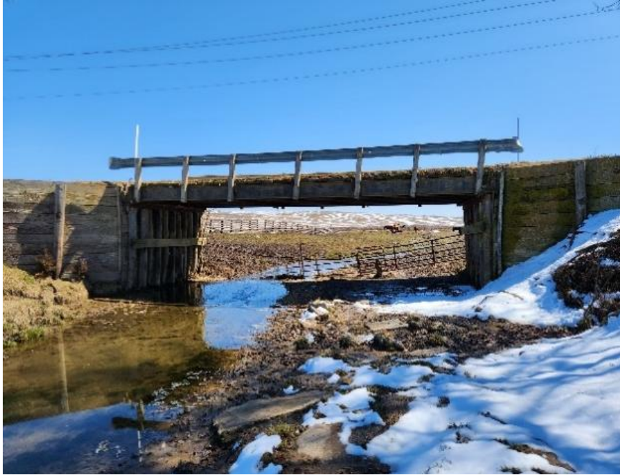
Figure 1: Jackson County – Bridge #15
